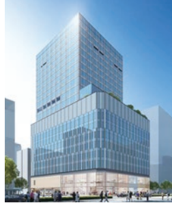
Sapporo Daibiru Building Three-function mixed-use building development Construction to be completed in April 2027
